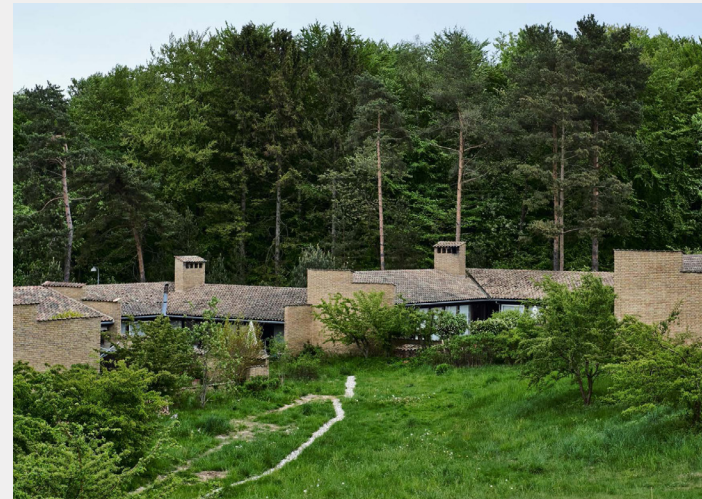
Kingo Houses, Fredensborg | architect Jorn Utzon
